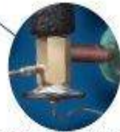
Thermostatic Expansion Valve (TXV)
